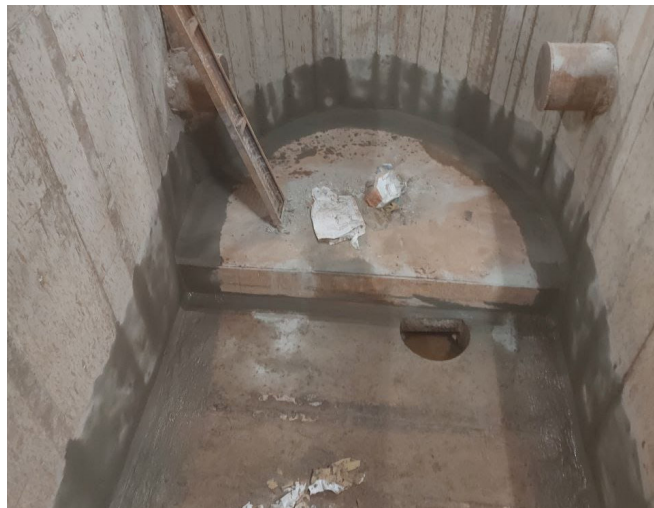
Corners chamfered with Xypex Patch'n Plug.
